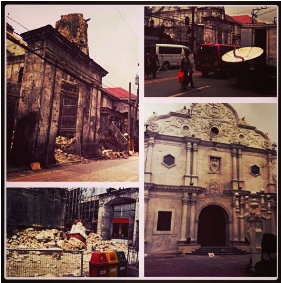
Earthquake damage in Cebu
